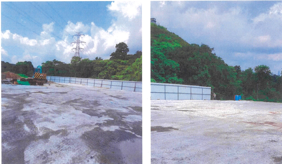
Figure 1b. The Application Site appears to be formed with concrete
